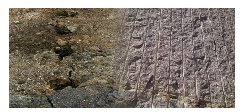
Besides the consistently applied production blasting performed in the mining and construction industries, controlled blasts and special custom blasts are needed for a variety of reasons including vibration and slope control. As Sarex Power Team we are proud to successfully complete and continue to provide services for special applications such as pre-split and smooth blasting in the mining, road construction, and dam and tunnel construction industries.
